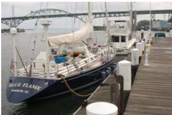
Yachts tie up alongside the bulkhead at Quality Yacht Services in Tiverton. The new marina will extend 300 feet from here out into Tiverton Basin and should be complete by next spring.
